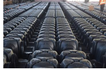
The CUPOLEX® - PONTEX® floor slab can be designed to be fully or partially suspended on piles, stem walls or grade beams. Additional reinforced internal PONTEX® rib beams provide a structure capable of spanning between foundations or piles.
