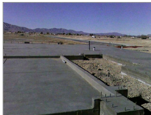
Finished Cupolex slab
