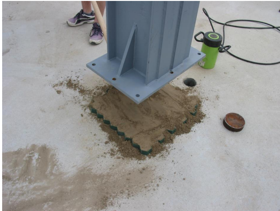
Fig. 2 Preparation of structure test
