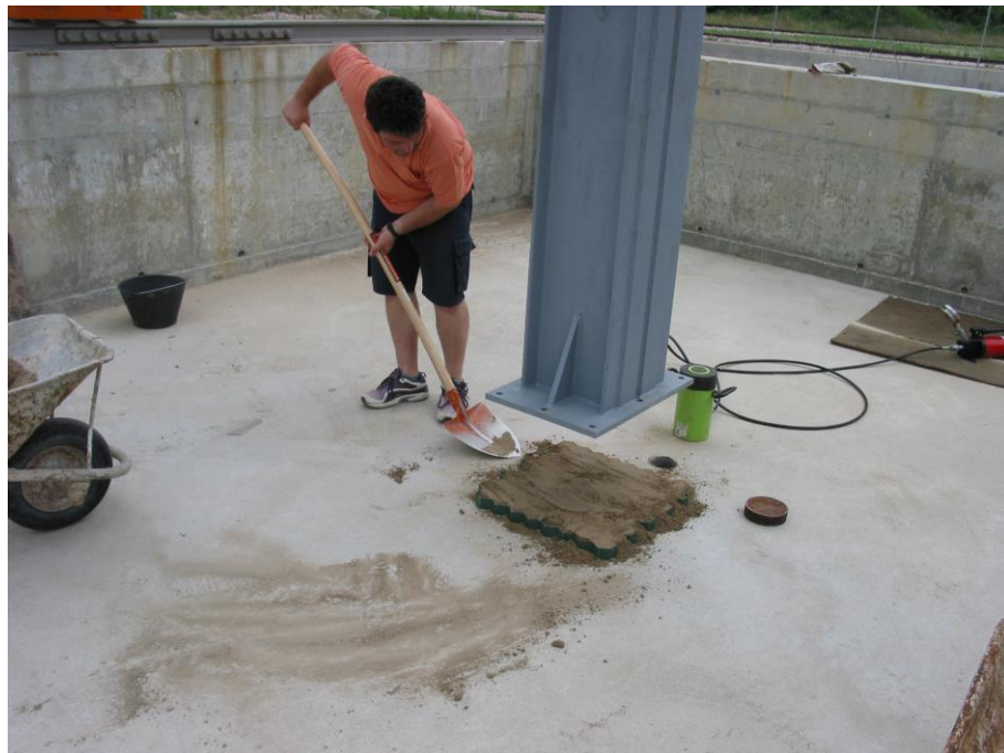
Fig. 1 Preparation of structure test
